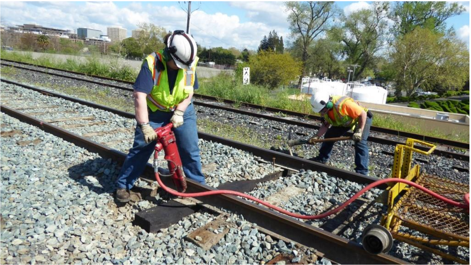
Heather drives spikes with the pneumatic spike driver as Joe digs under the end of a tie so that the nipper-bar can get beneath it
