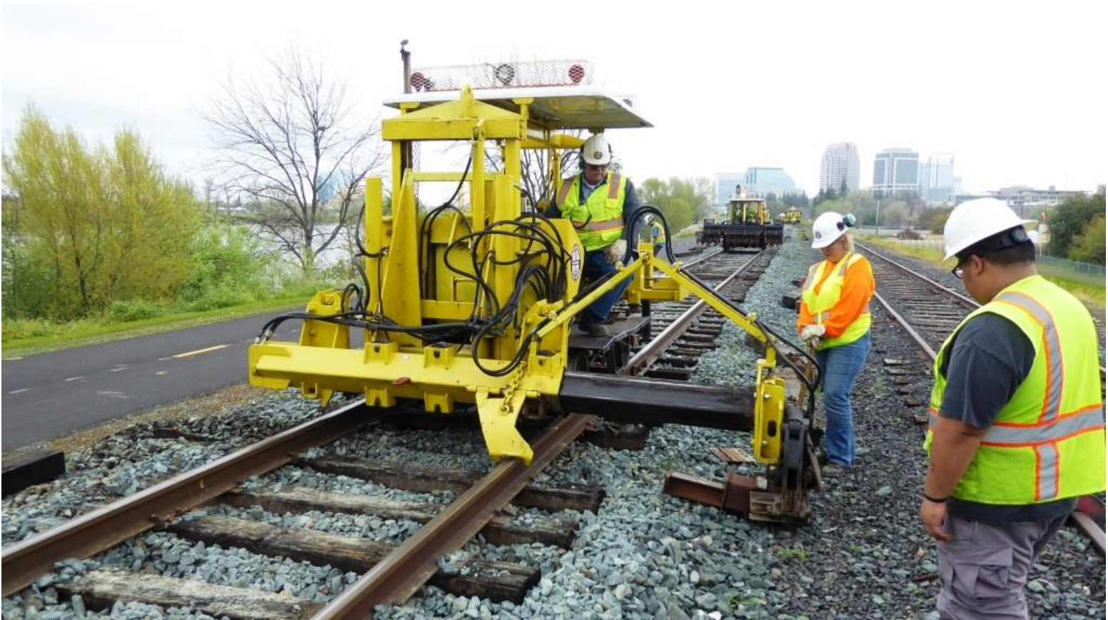
Bev and Anthony get the ram-attachment set up on the Jackson 125 for Chris to push a couple ties out
