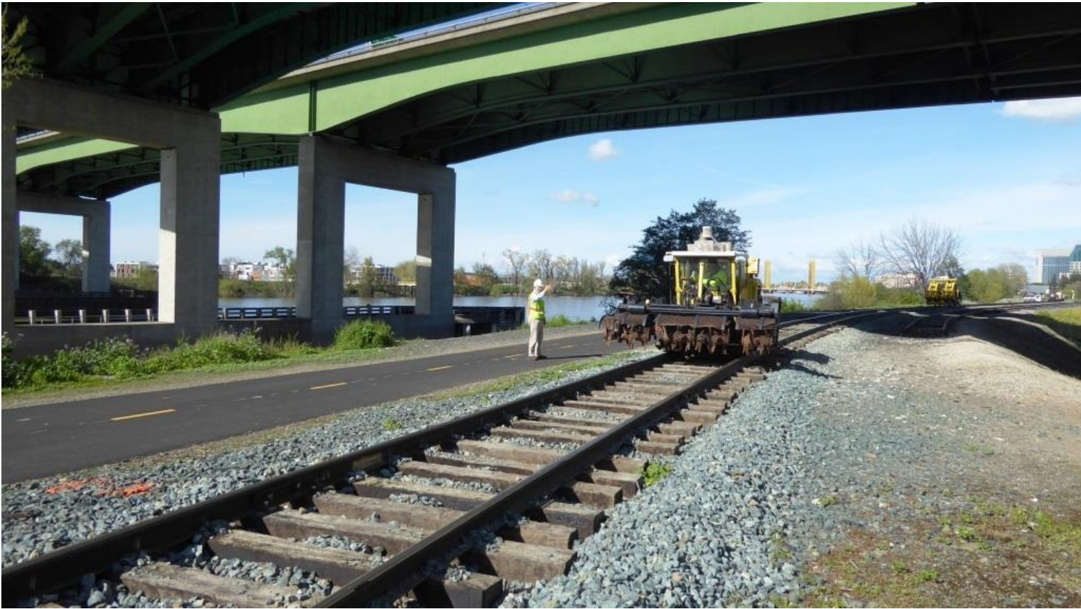
Signals Paul waves to Alan in the scarifier as he clears the circuit
