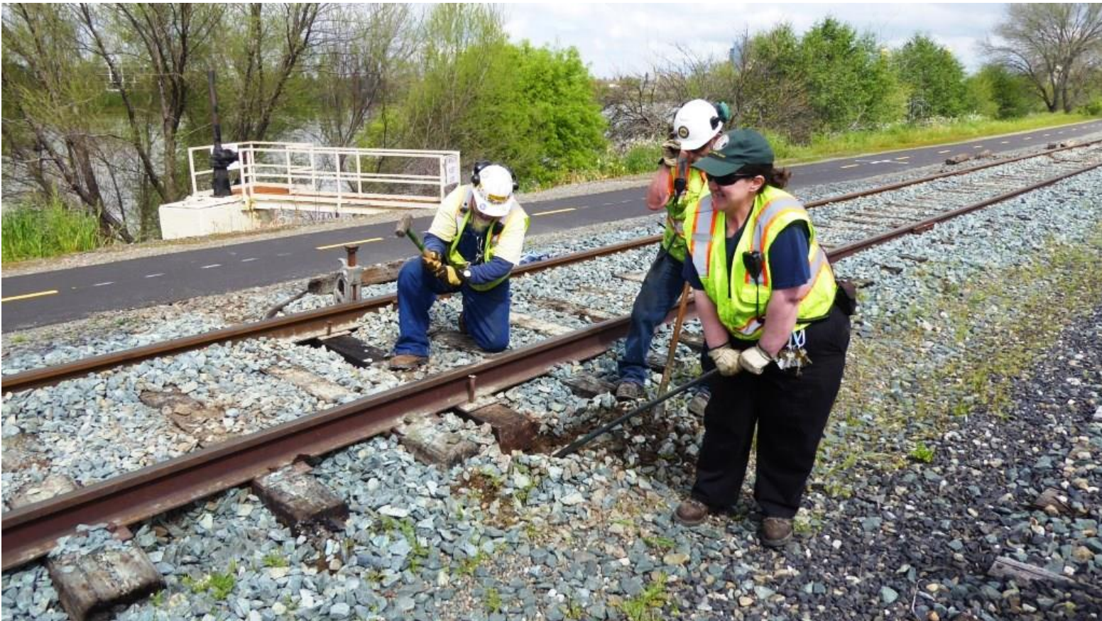
Heather nips-up the tie as Mike F. sets spikes
