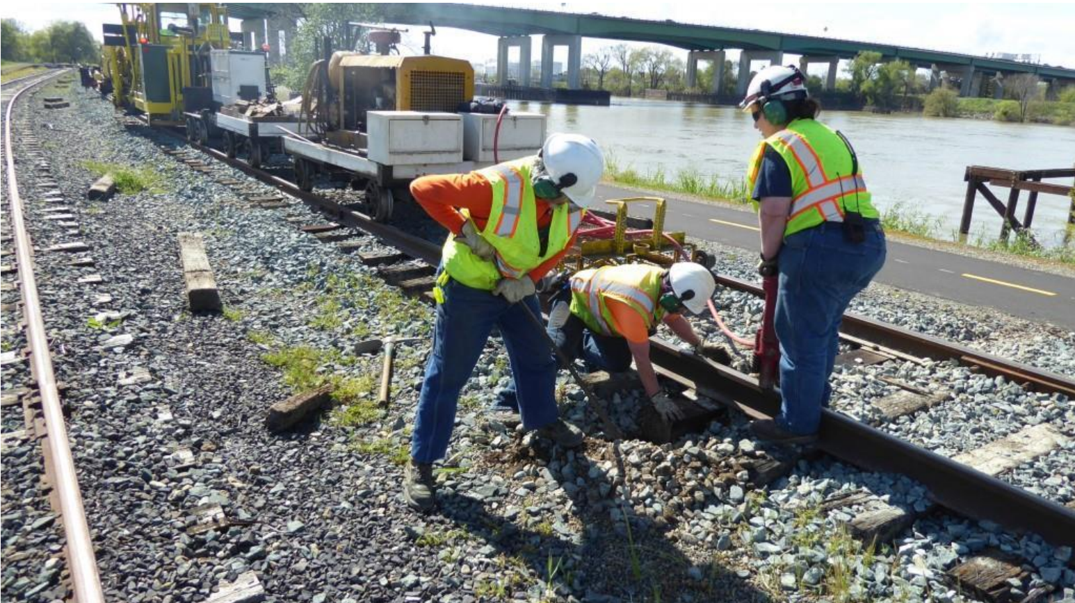
Ed nips-up the tie as Joe re-sets a spike that fell out. Heather stands by with the spiker
