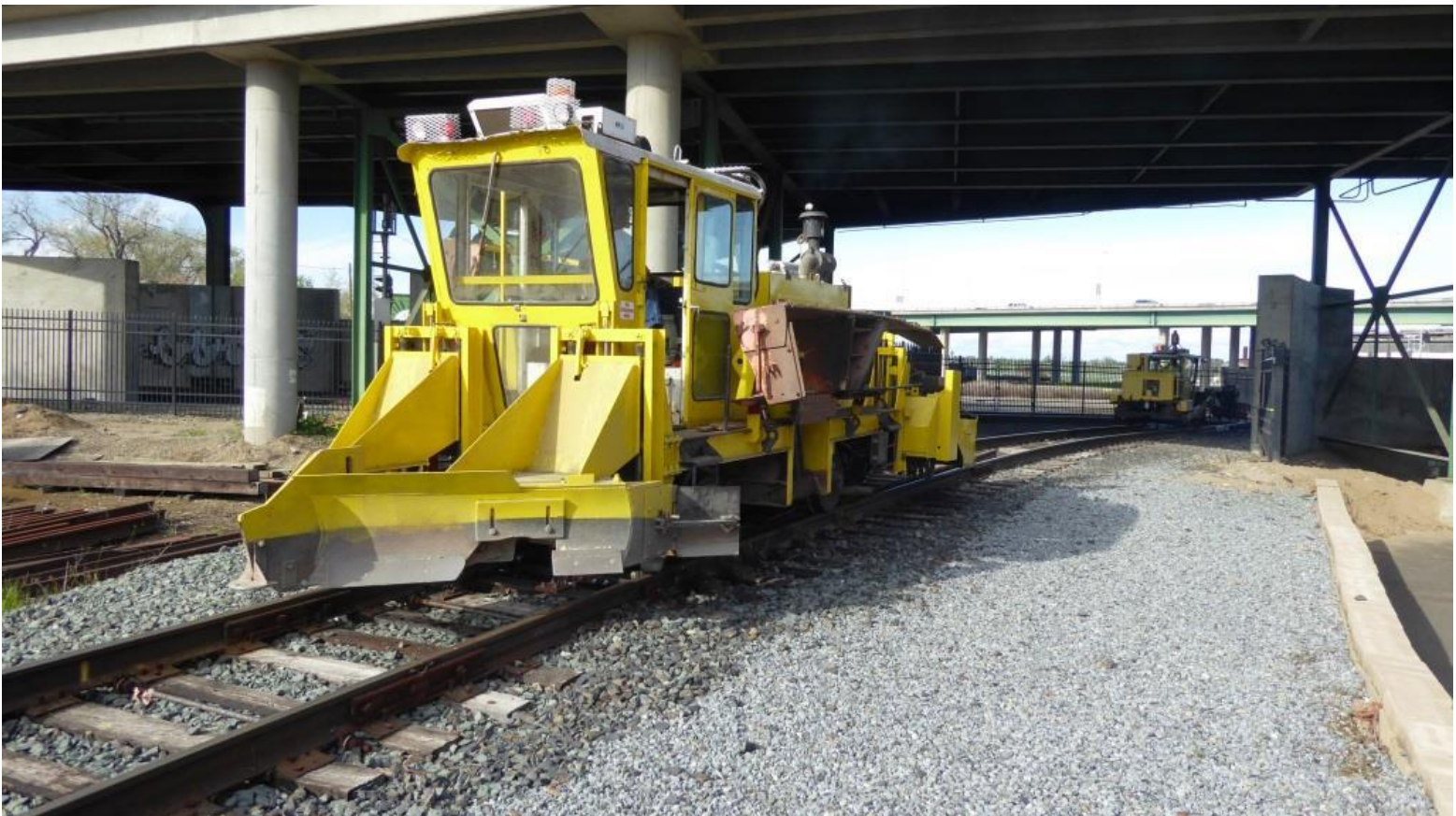
Heading home: at the end of the day, the scarifier and regulator return to the Shops over the UP Main
