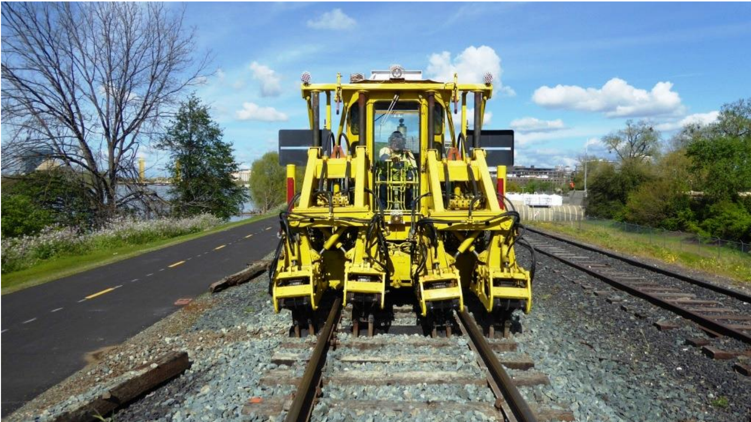
Mike F. brings in the tamper and tamps the new ties
