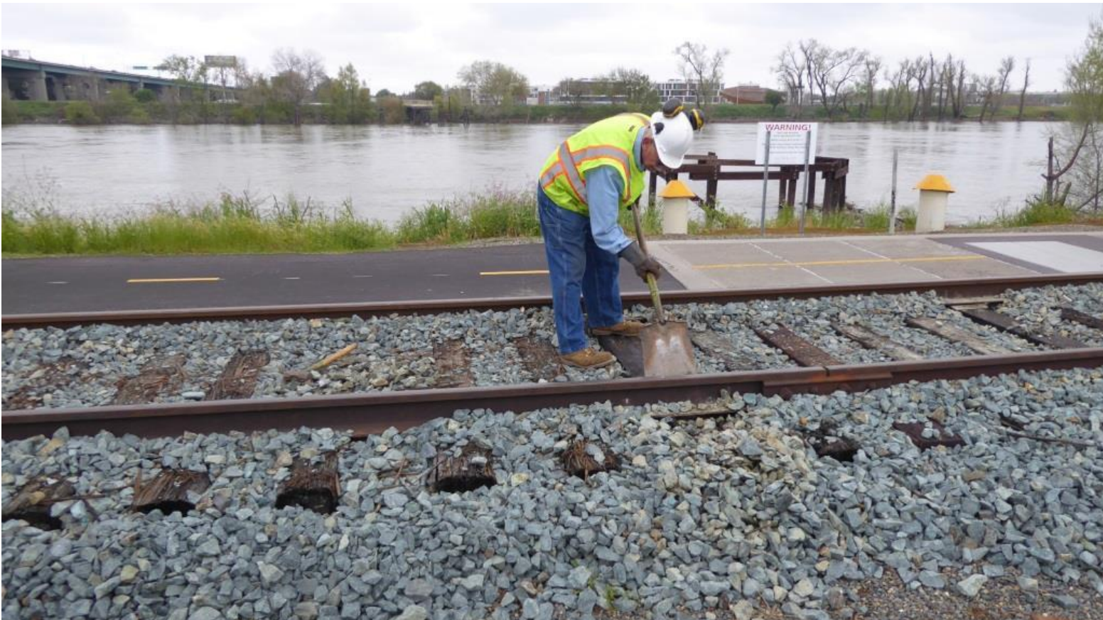
Clem fills rock in around the ties
