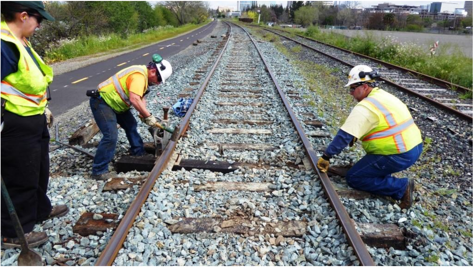
Joe and Mike F. place tie-plates and set spikes
