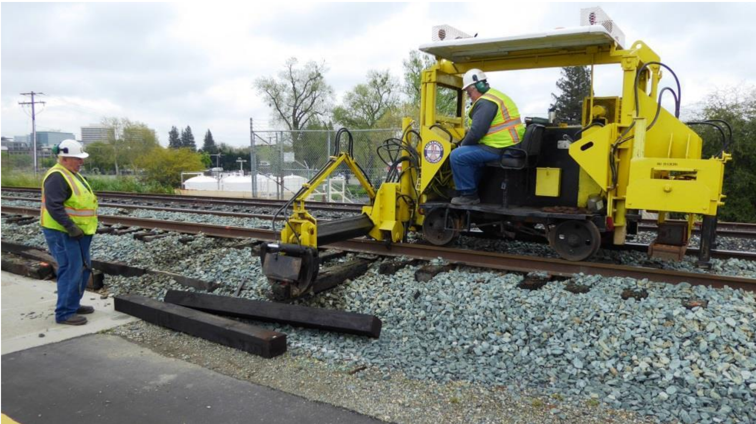
Chris, on the Jackson 125 tie-exchanger, pulls an old rotten tie out...
