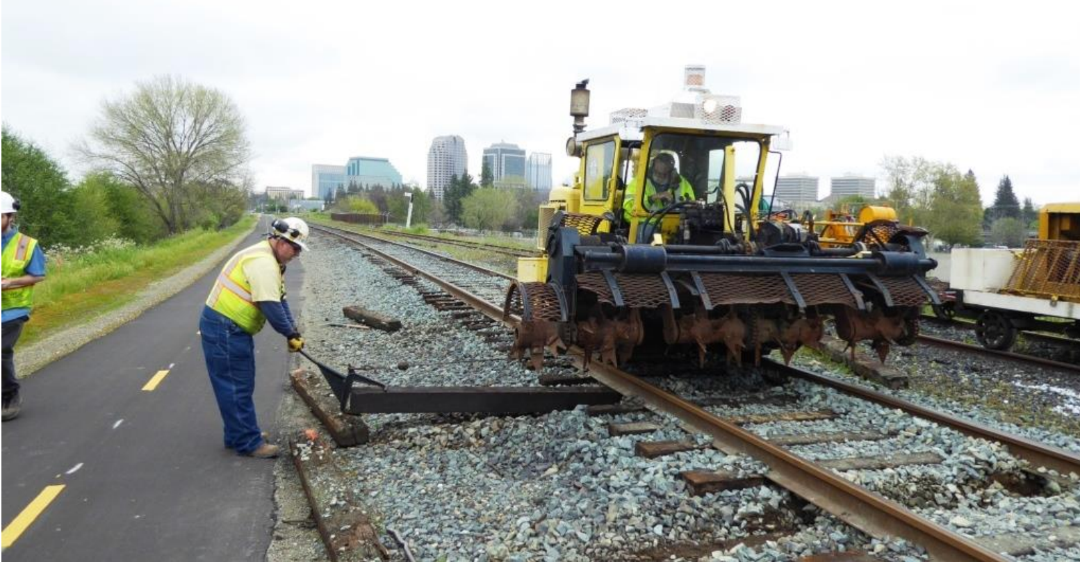
Alan in the scarifier-inserter pulls a new tie under the rails as guided by Mike F.
